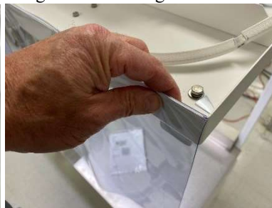
9. a back-cut at the hem allows the fascia and curtain to be better aligned with the end of the ceiling as shown
