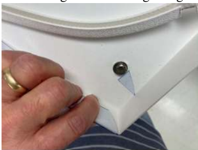
9. a back-cut at the hem allows the fascia and curtain to be better aligned with the end of the ceiling as shown
