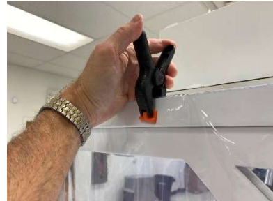
8. HINT : using a small spring-clamp near the ends helps keep the fascia/curtain from falling while working along the length of the ceiling
